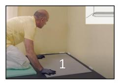
Start with a first, full length tile (n°1), which comes in the top left corner of your room. Preferably lay the 2 sides with tongue towards the walls and make sure that the expansion joint of 5 mm is respected. The groove or tongue is not part of the expansion joint. Cut them off if necessary.
